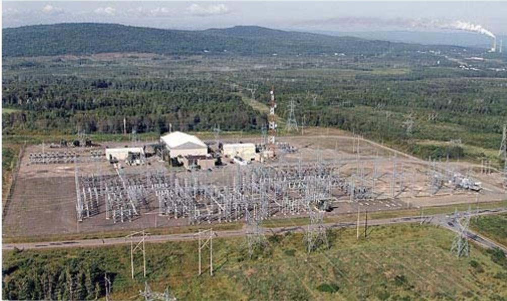
**Fredericton, N.B.** – NB Power has awarded a contract to ABB Inc. to begin investing 30 million dollars in an upgrade to the Eel River High-Voltage Direct Current (HVDC) Converter Station, located near Dalhousie, NB (pictured above). The bidirectional station transfers up to 350 megawatts (MW) of power and is one of the two facilities that allows for power exchange between New Brunswick and Québec, providing access to Maritime and New England markets.
