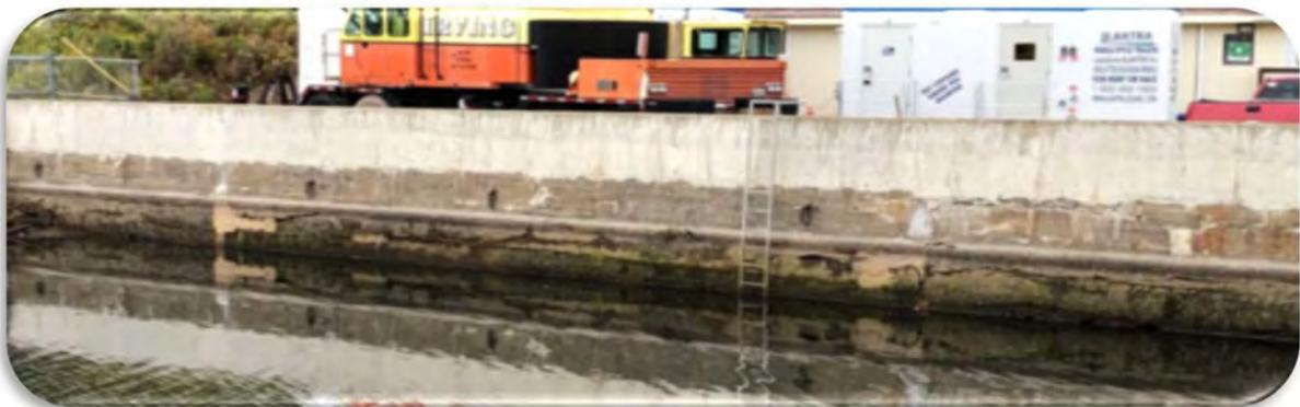
**Photo 7: Photograph Showing the Deteriorating Condition of the Concrete Walls in the Forebay Area**
