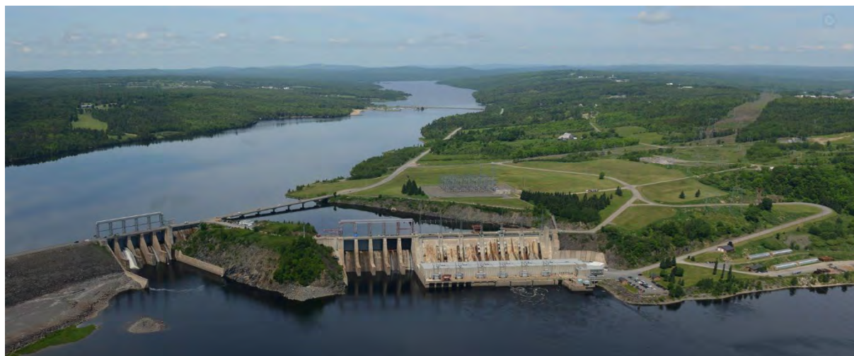
Figure 8.2: Mactaquac Generating Station
