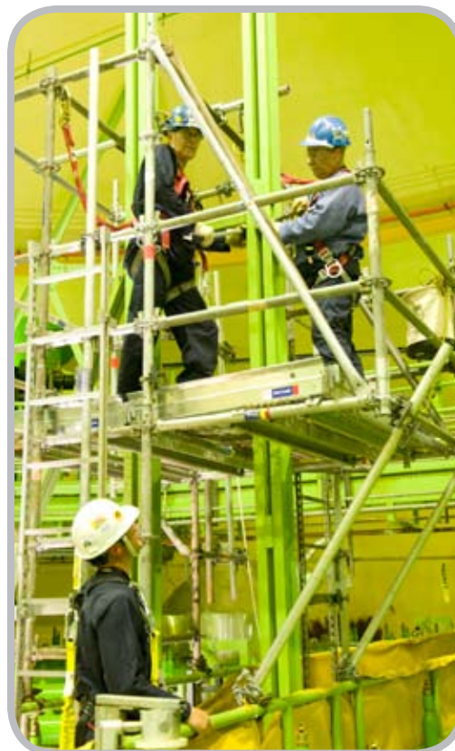
Employees work on scaffolding at the Point Lepreau Generating Station.
