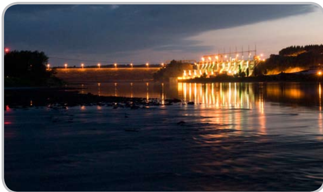
The Mactaquac Generating Station.
