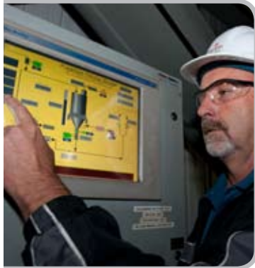
Roger Fowler, Shift Supervisor at Coleson Cove Generating Station, makes an adjustment to the controls on the petroleum coke pulverizer.
