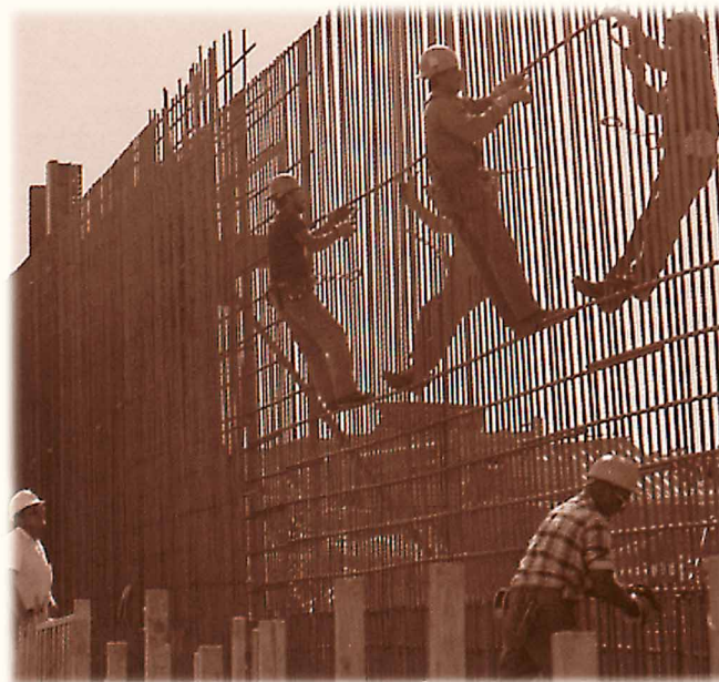
Belledune generating station under construction, 1990
