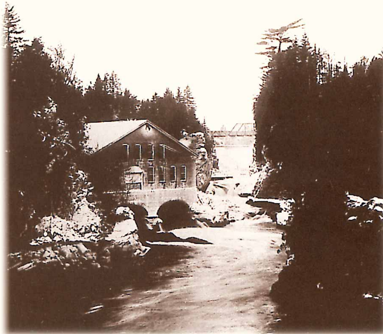
Pulp and paper company power plan, St. George, circa 1905 (National Archives of Canada, PA 41747)
